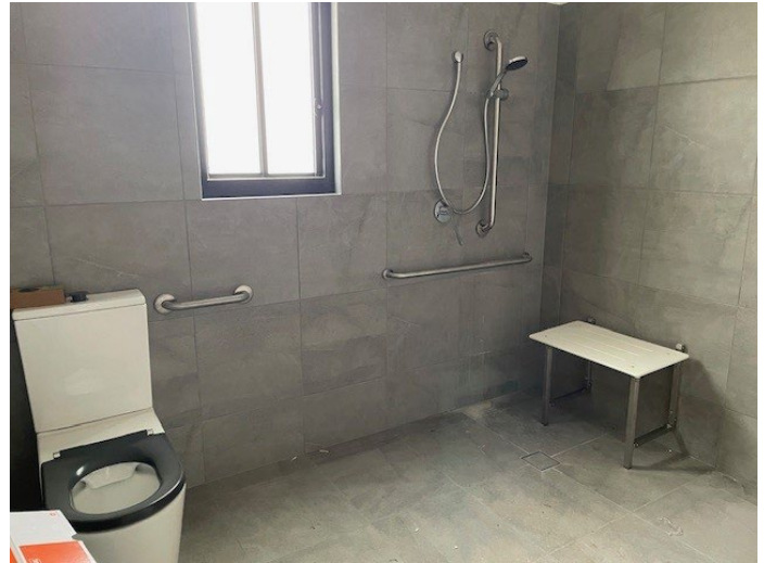
Office building – disabled facilities
