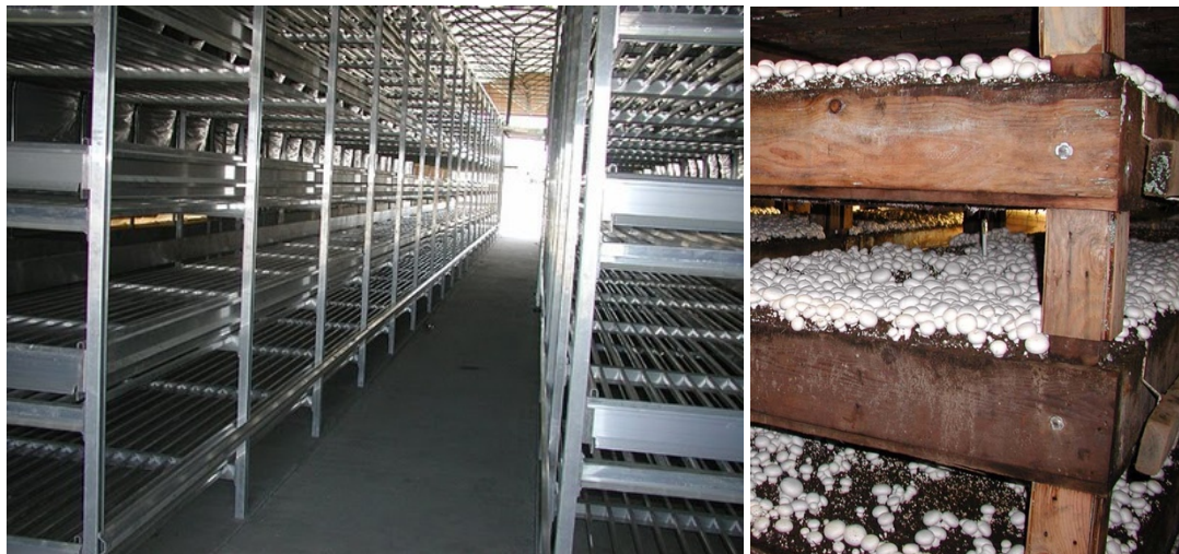
Figure 47. Galvanised belt and shelf systems allow more efficient cook-out than older tray systems
