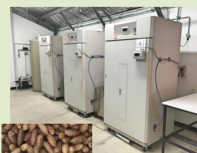
Q-fly pupae were stored at the Plant Growth Facility at Macquarie University in Sydney
